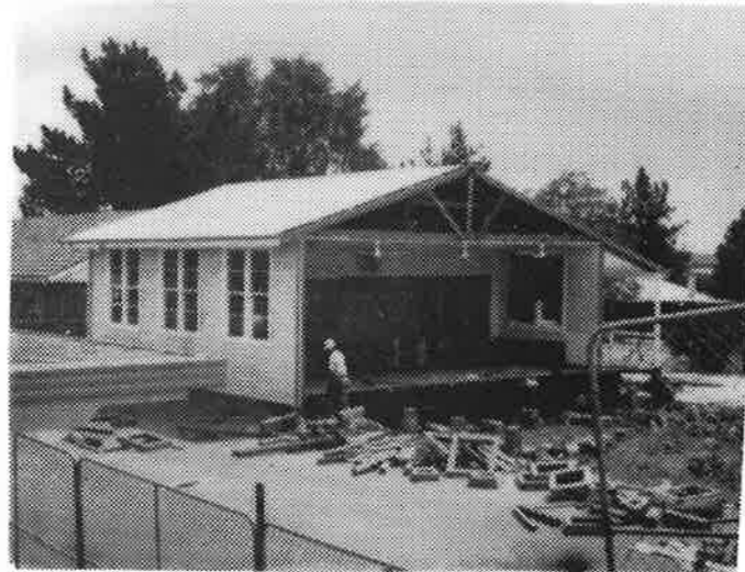
The 1953 weather board building was cut in half, lifted by cranes, swung around and resituated on brick piles. After being brick veneered, it became the present Administration area.
